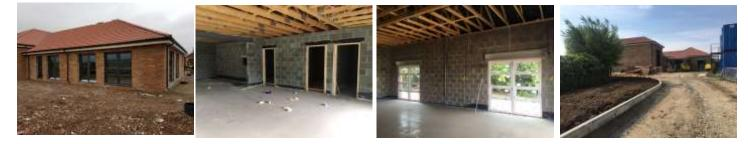
During the past couple of months roof tiling works have been completed, along with the installation of windows and doors. This has provided a water tight building, allowing for the floor screed to be laid and mechanical/electrical/joinery first fixes to be completed.
